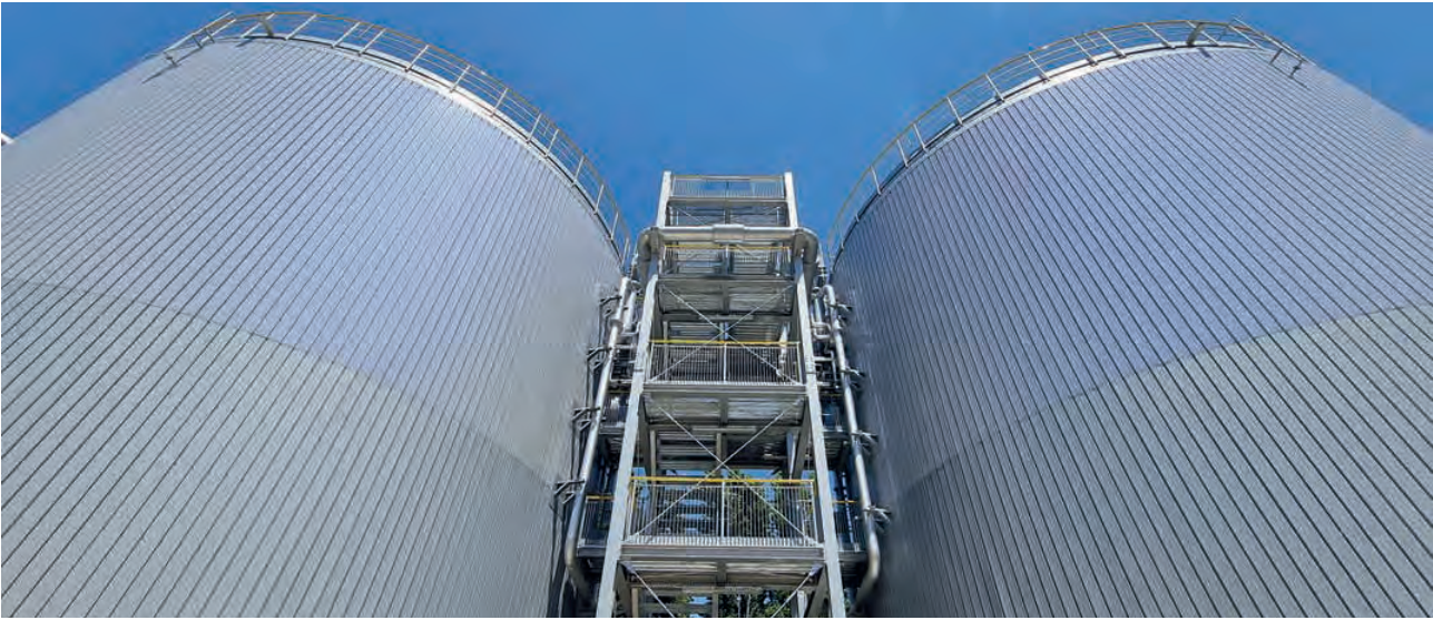
Two thermal storage tanks, each with a capacity of 2,200 m 3 , have been built at the Centrale Nord power plant site in Brescia, Italy
