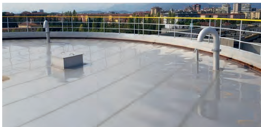
Figure 3. The stainless-steel membrane cover is a self-supporting, lightweight construction with high mechanical strength that can withstand snow loads and strong winds. It is prefabricated in the factory, transported to the construction site, and installed on site
