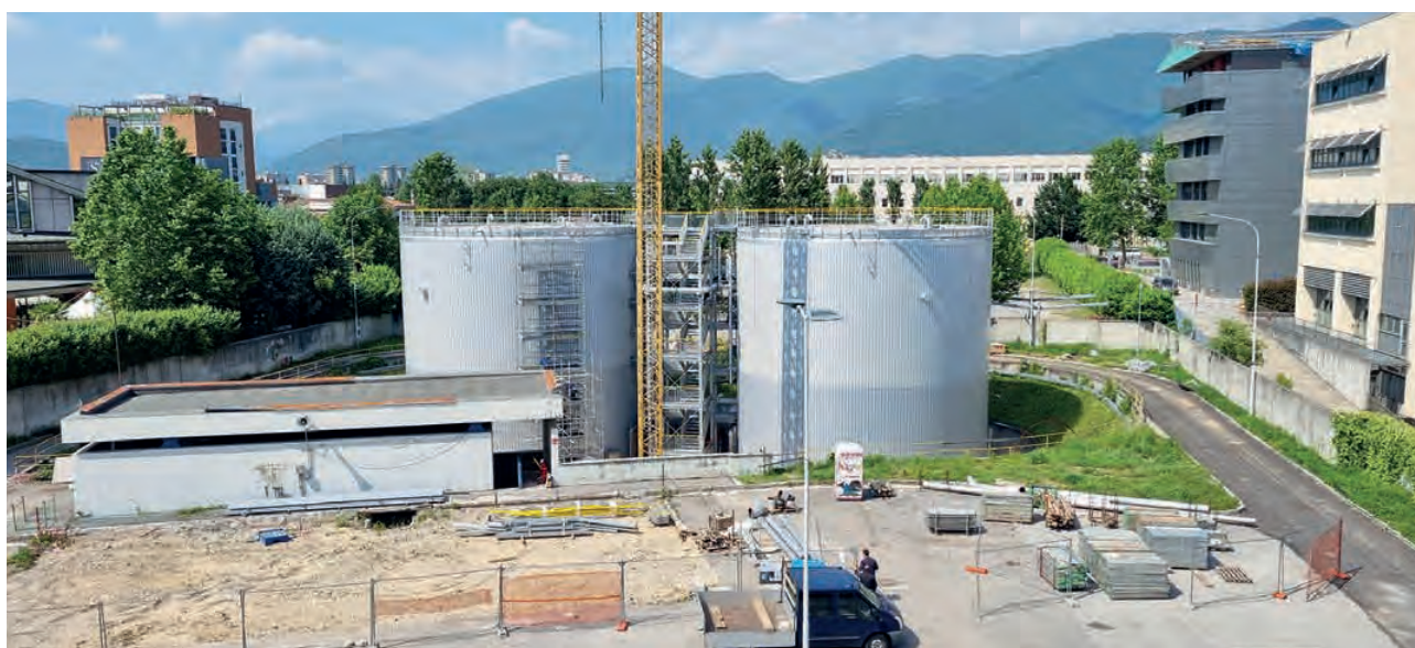
Figure 4. Lipp welding technology was used to construct two thermal storage tanks at the Centrale Nord power plant site
